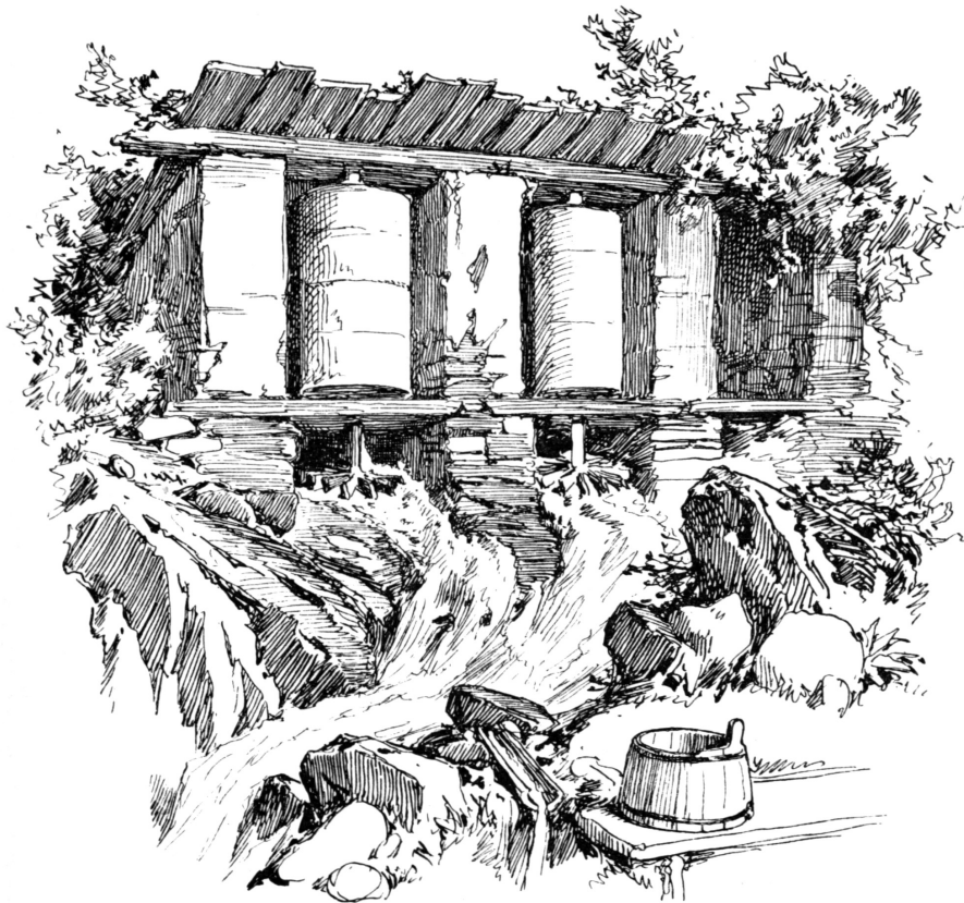
3: Fig. 2. — Praying-barrels propelled by water-wheels, at Soonum. From a Sketch by the Author.
